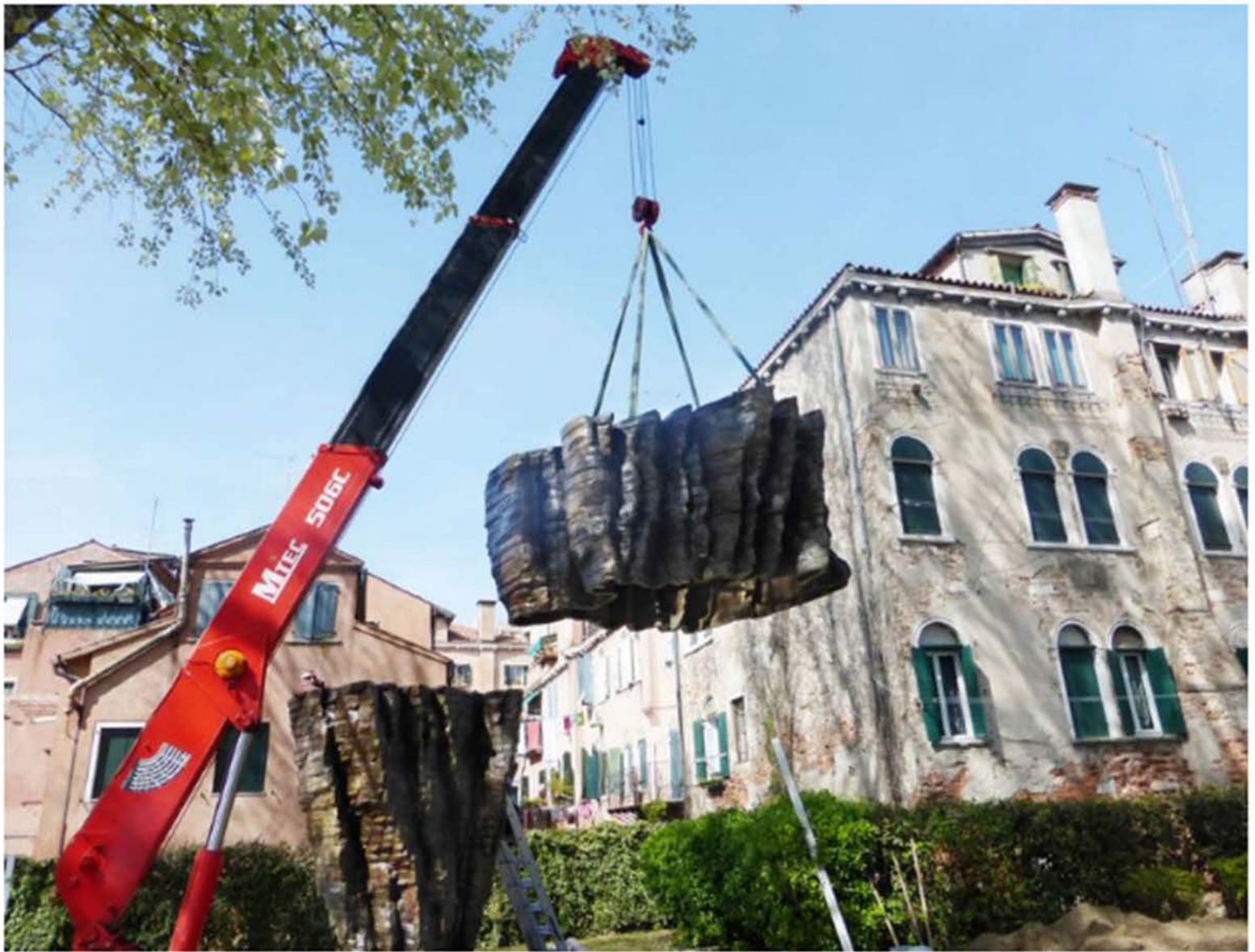
Adding the middle section of Bronze Bowl with Lace , a bronze statue that weighs close to eight tons. Source: Yorkshire Sculpture Park via Bloomberg
